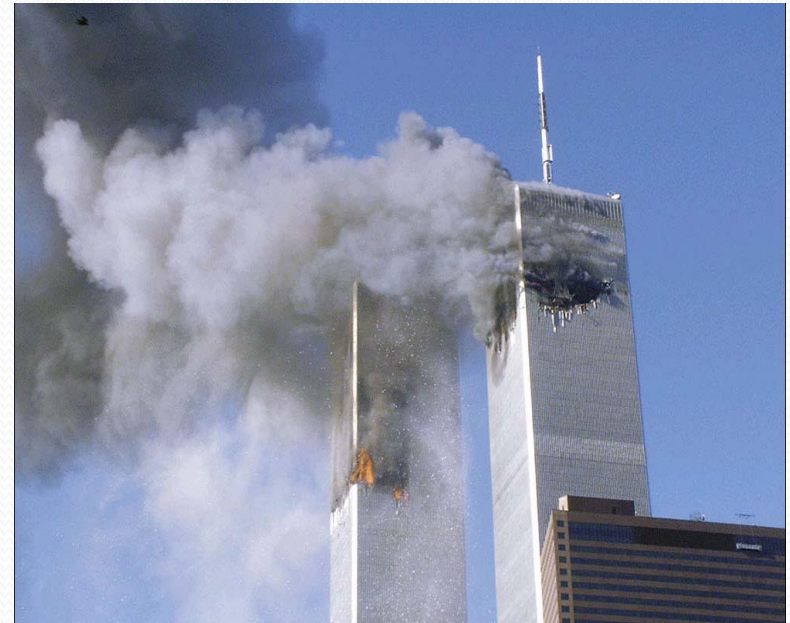
Damaged and Burning WTC 1 (right) and WTC 2 (left) on Sept. 11, 2001
