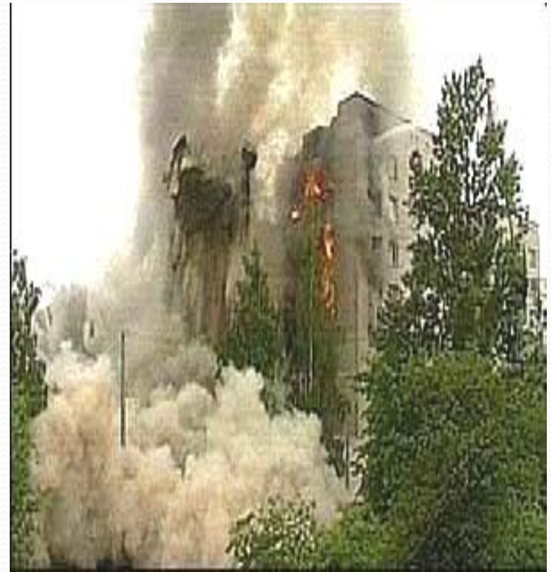
Collapse of St. Petersburg Apartment Block (Bietel & Iwankiw, 2002)
